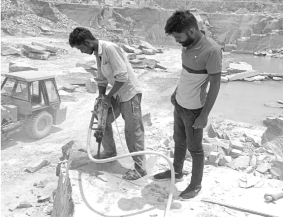
Drilling work in progress in one of the mining sites
